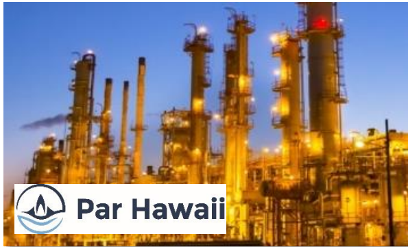
Refinery renewable integration
